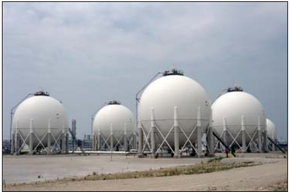
Aux Sable's Channahon, Illinois, facility has nine storage tanks that have the capacity to store 200,000 barrels of natural gas liquids.
