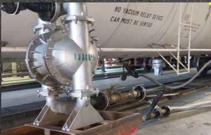
Pump to offload effluent for filtration process
