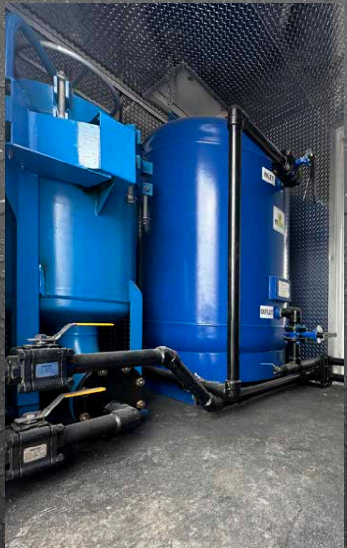
Three part water filtration system and holding tanks for tank car cleaning
